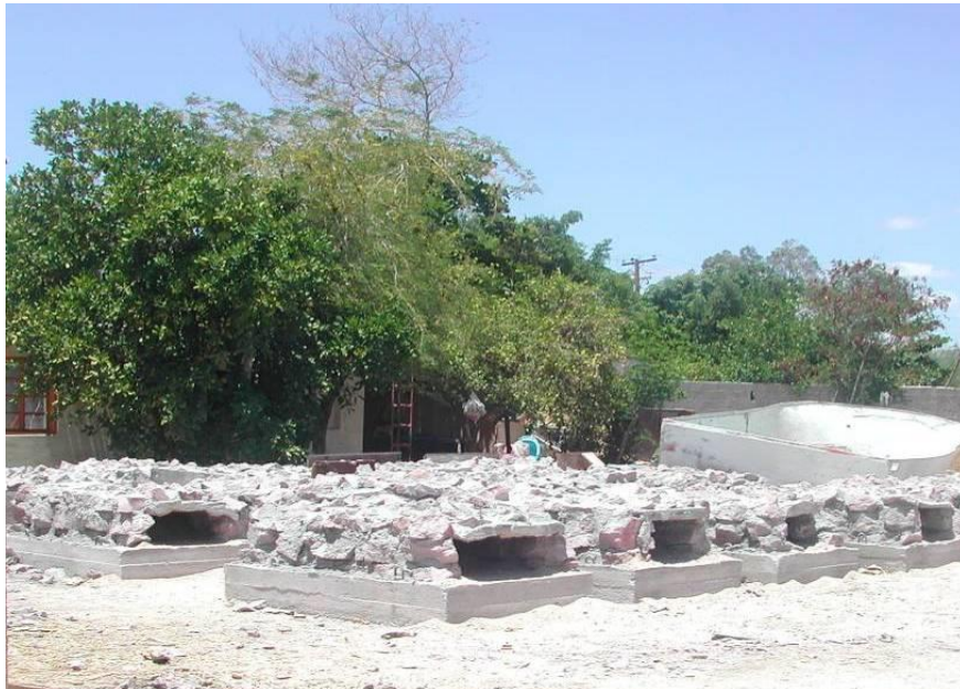
Photograph 3. Habitat modules immediately following construction awaiting deployment.
