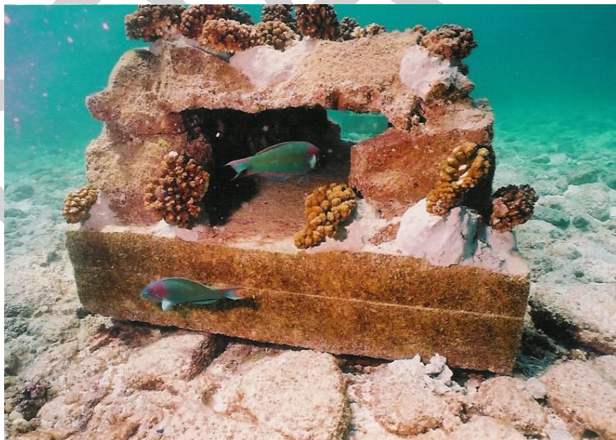
Photograph 6. Close-up view of habitat module showing the opening that extends through the center of the module. Recently re-attached corals are also visible on the module.
